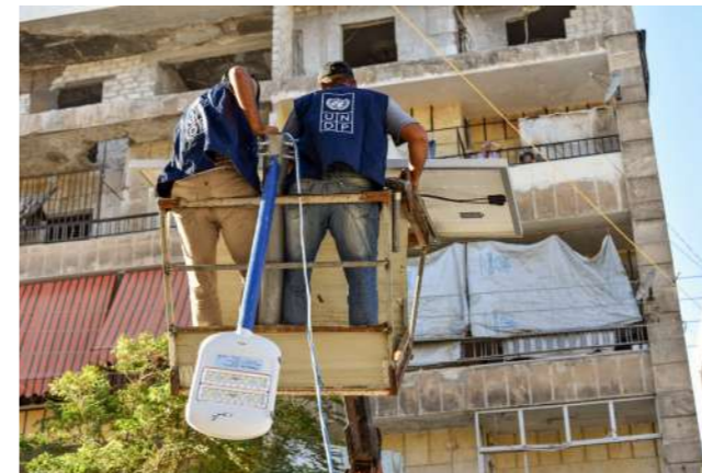
Rehabilitation of an electricity network in Al-Hassakeh Governorate
