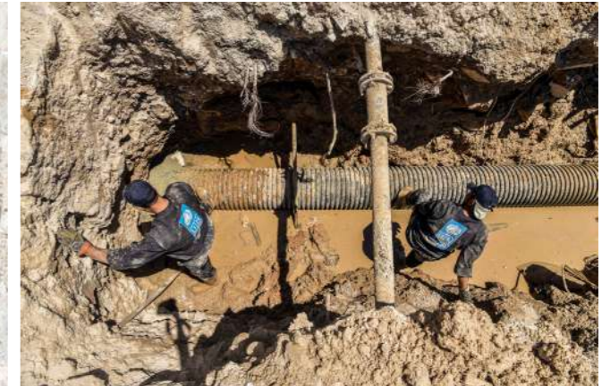
Sewage network rehabilitation works in Aleppo city
