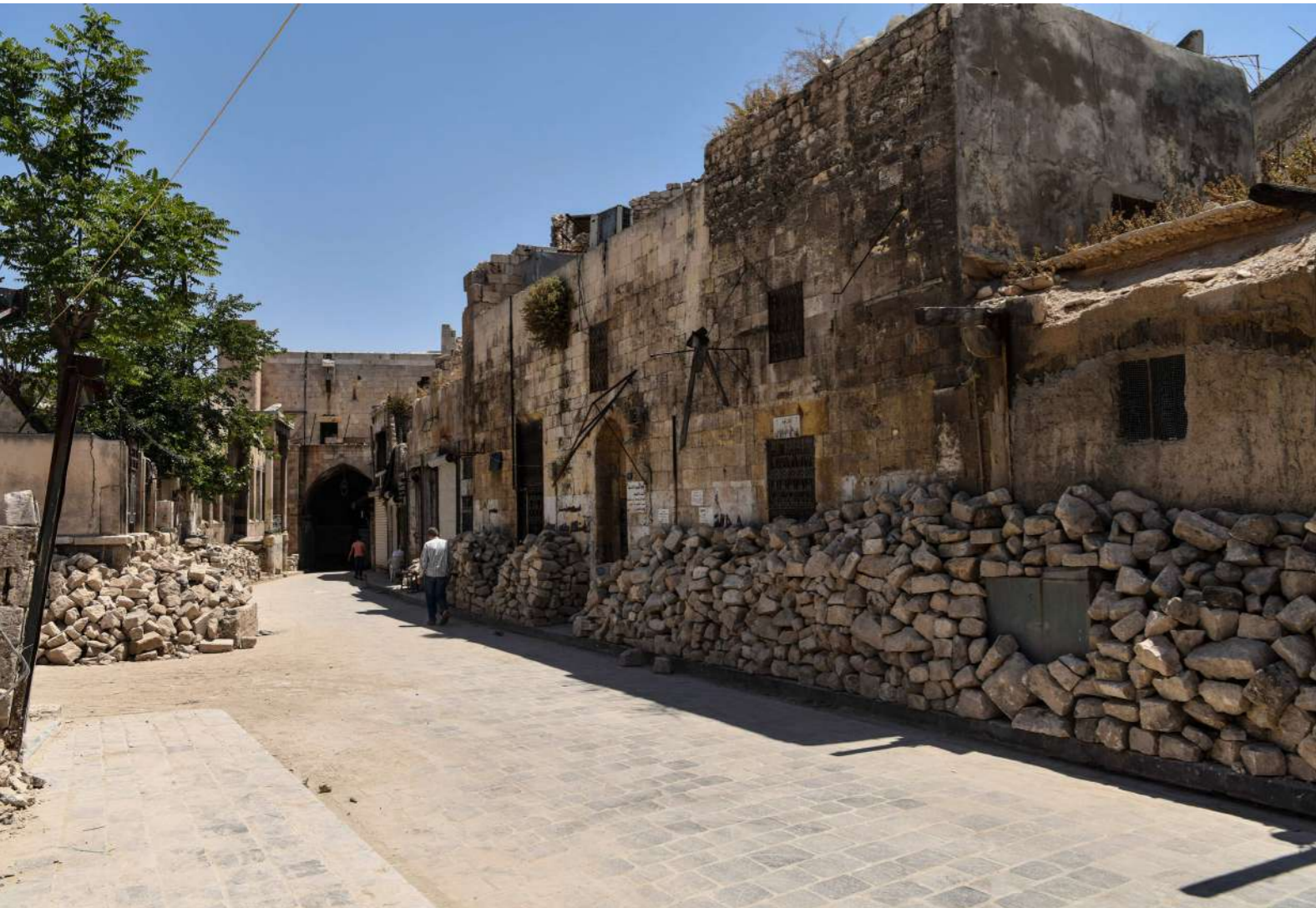
Old stones sorted out of the debris that were removed from Bab Al-Hadid neighbourhood and collected on site to be reused in future rehabilitation works of the same neighbourhood, Old city of Aleppo ©UNDP-Syria
