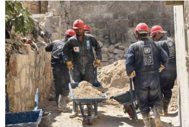
Rehabilitation works of a water network in Aleppo
