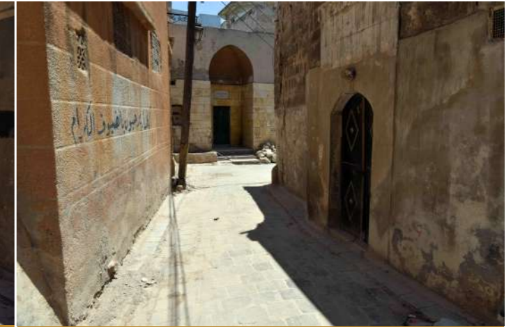
Neighbourhood in Old Aleppo cleared of debris with the support of UNDP ©UNDP-Syria
