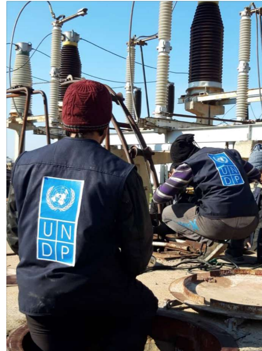
Rehabilitation works in Al-Tabqa hydroelectric plant in Ar-Raqqa Governorate ©UNDP-Syria
