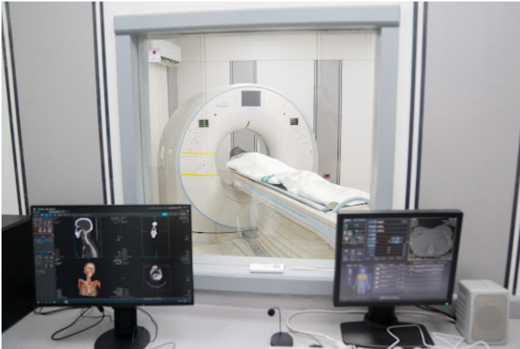
CT scanner installed at Al Tal Hospital in Rural Damascus @UNOPS 2022
